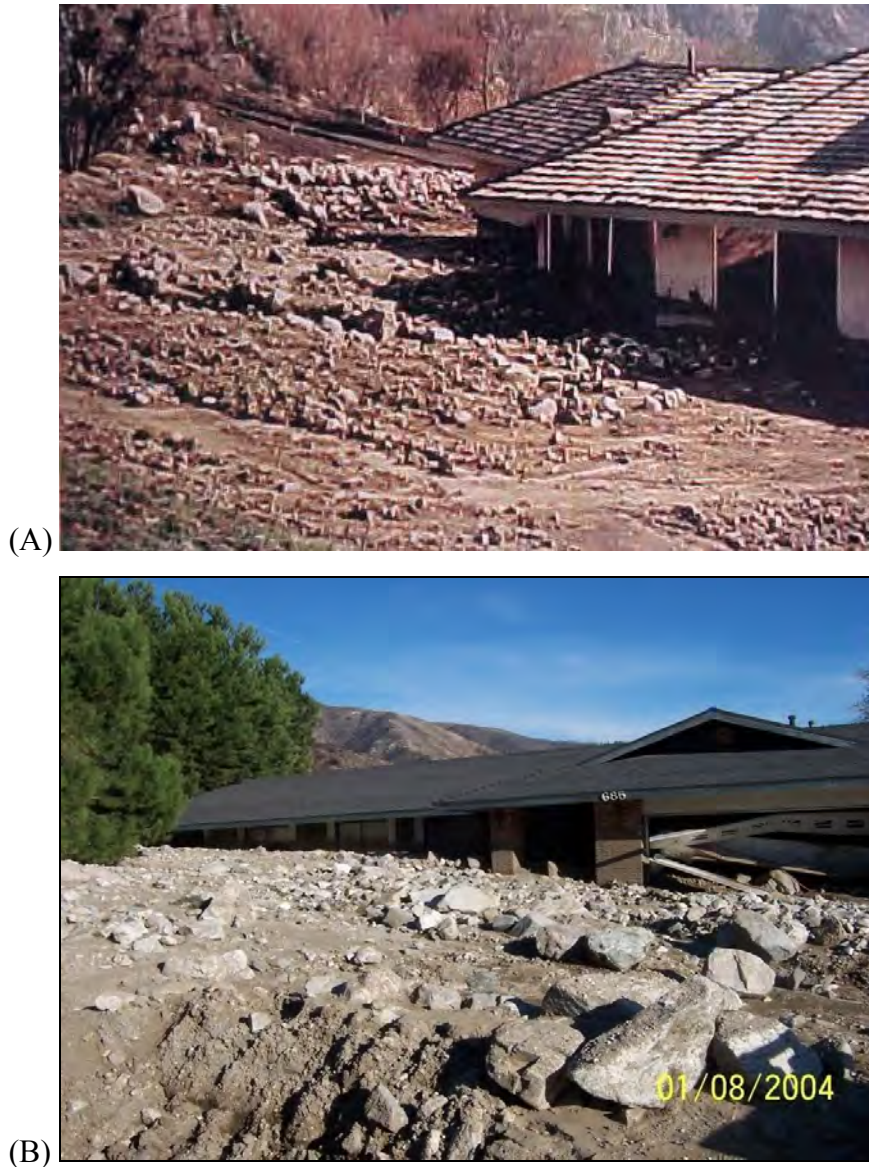
Figure 2. Debris-flow damage to homes in (A) Glencoe Heights along the San Gabriel mountain front in response to January 1969 storm (LADPW photograph), and (B) Devore along the San Bernardino mountain front following December 2003 storm (U.S. Geological Survey photograph).
